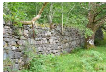
Photograph 5: First impressions are that this is a drystone wall; only on closer inspection is a recessed lime/cement mortar evident. I am guessing that this may be the original boundary between Achnacarry and
